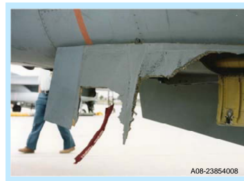
Figure 8 F-16 Ventral fin Damage on First Test Flight With LANTIRN Pods (Ref. 24)
